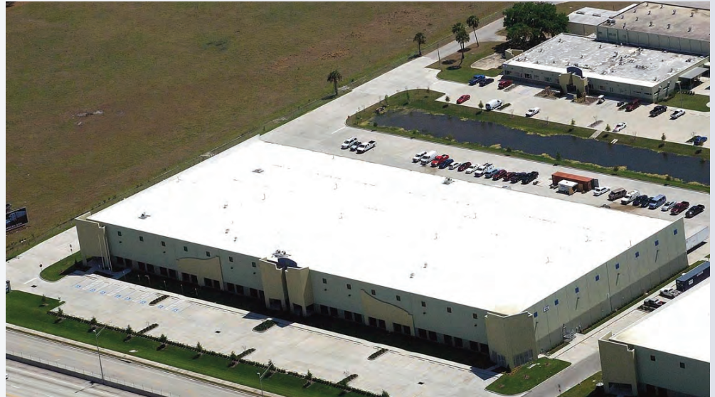
GTECH's new 98,000 square foot facility in Lakeland, FL. (photo courtesy of Aero Photo)
