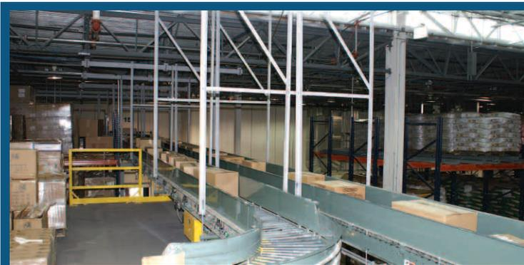
*A Hytrol ABEZ Zero Pressure conveyor shown exiting the third level of the two pick modules in order to bring cases to shipping.*
