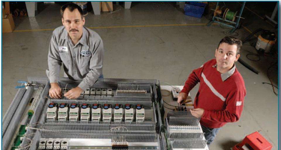
TriFactor's Bill Waikem and Todd Bixby assemble the back panel of a UL508A industrial control panel. This will get mounted inside the steel cabinet and will be used to process signals from sensors in order to properly control all of the motors in the conveyor system and transfer information about product on the conveyor system to the customer's ERP system.
